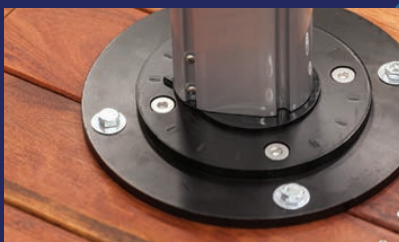
Figure C Align the indicator arrow with a notch
